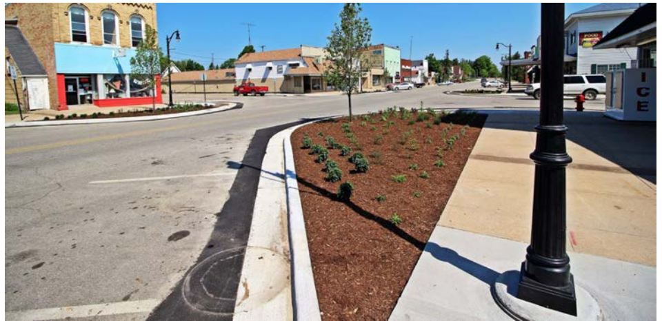
A landscaped bulb-out shortens the distance a pedestrian has to cross the street, making the trip safer and more enjoyable
