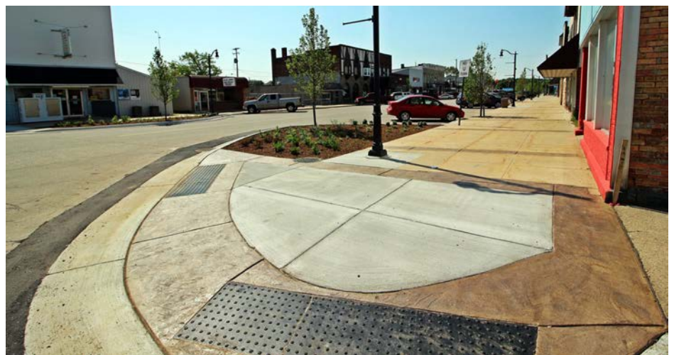
A landscaped bulb-out is seen in the background, the textured sloped curb cut is designed for blind pedestrians and wheel chairs
