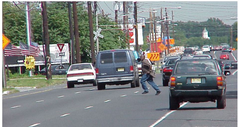
With lack of crosswalks, pedestrians dangerously run through busy traffic to reach their destinations
