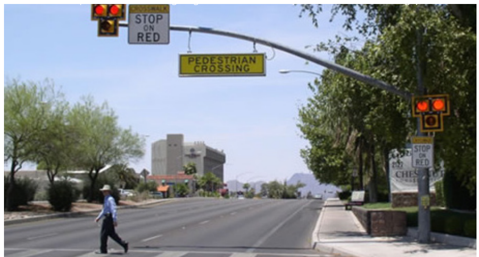
The Federal Highway Administration endorses crossings with beacons on major arterials to keep pedestrians safe
